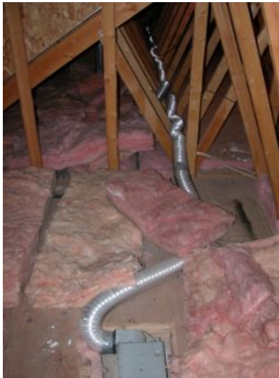
Bath fan vents appropriately vented to exterior.
