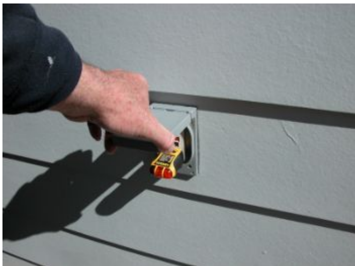
Proper exterior GFCI outlet shows functional
