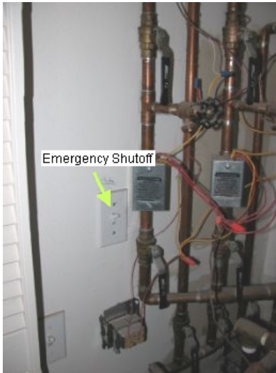
Boiler shutoff
