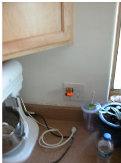
Ground fault circuit protected.
