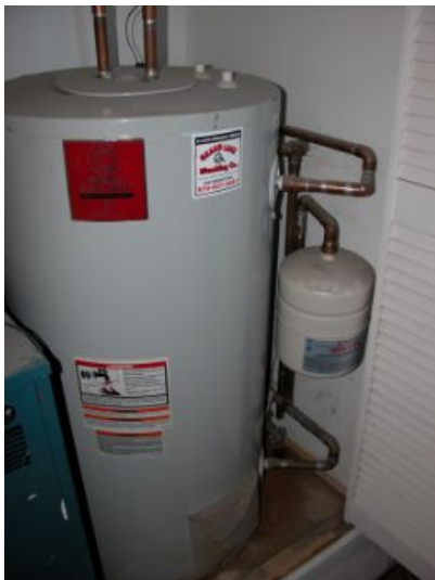
WH at end of life, recommend replacement, decouple from radiant.
