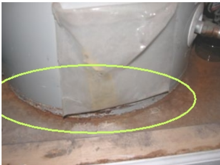
Water Heater show signs of rust/age, water stain on base.
