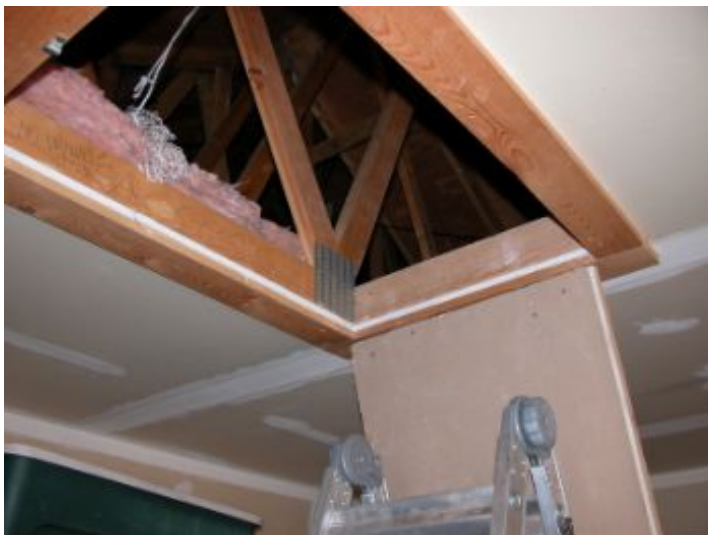
Primary attic access reveals insulated garage ceiling.
