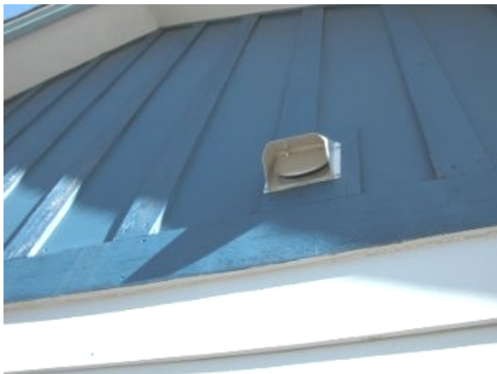
Paint in good shape, external dryer vent functional.
