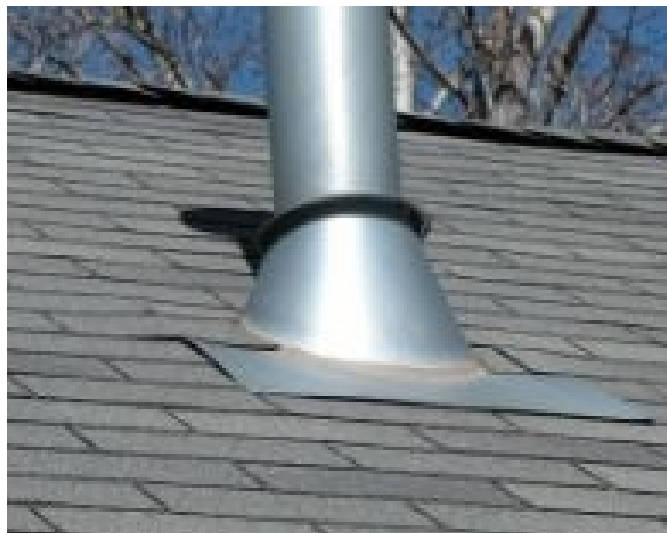
Flue stack properly flashed.
