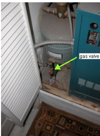
Main Boiler Gas Shutoff.
