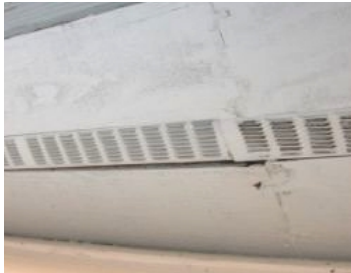
Area of soffet needing maintenance caulking.
