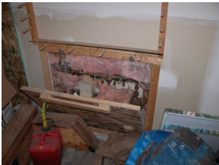
Primary water entrance panel from garage. Proper insulation.
