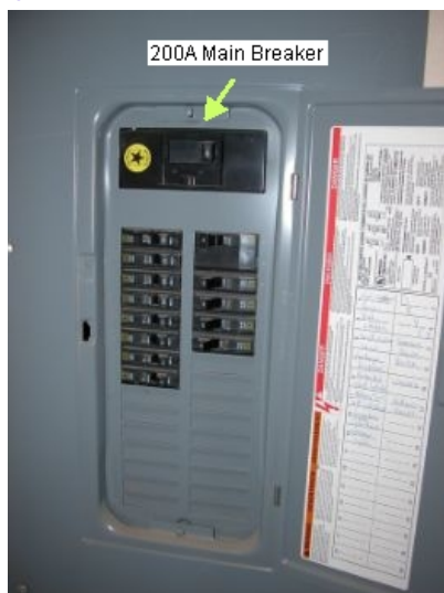
Clean well-mark QO Service panel with expansion slots.
