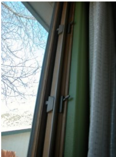
Some window-latch adjustment needed.
