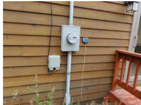
Meter is firmly attached.
