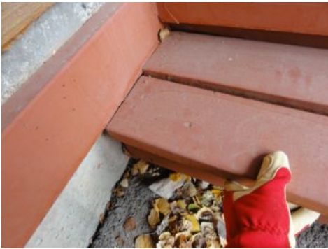
The step is loose and should be repaired. Trip hazard.
