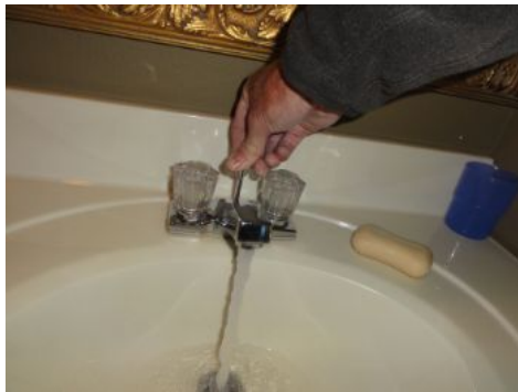
Drain stop non functional on this sink.
