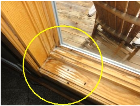
Water damage on this particular window
