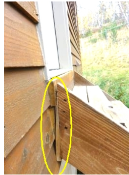
Step stringers are pulling from wall.
