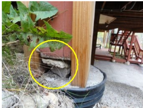
Deck pier is supported by concrete shards. This bears weight of jacuzzi/deck. The 2x's help displace load.
