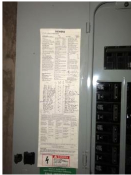
This panel is at full capacity.
