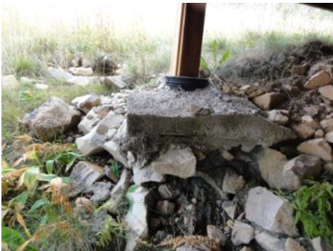
This deck pier is improperly designed, it supports jacuzzi weight.
