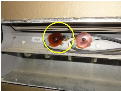
Heater on right side of lower pellet stove is not operating. Signs of scorching on wiring.
