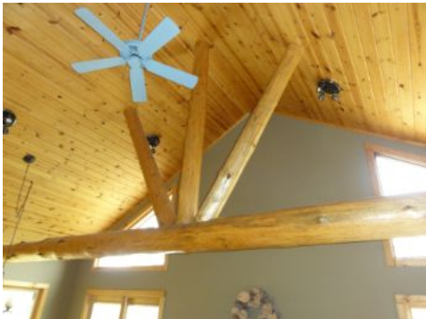
Log truss system in living area cathedral ceiling.
