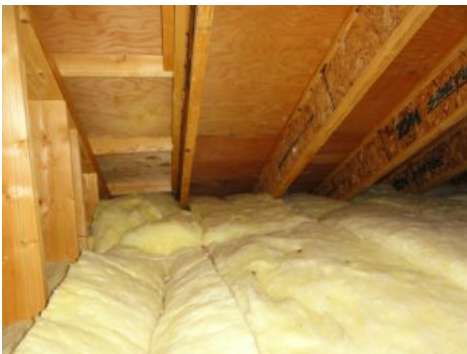
No insulation baffles at soffits block air flow.
