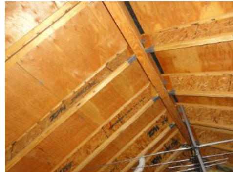
Engineered I beam truss system here. No signs of moisture intrusion.
