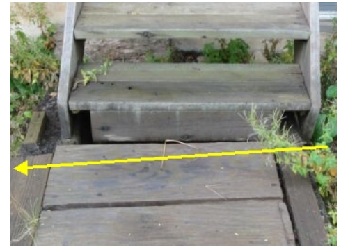
Landing is moving with erosion.
