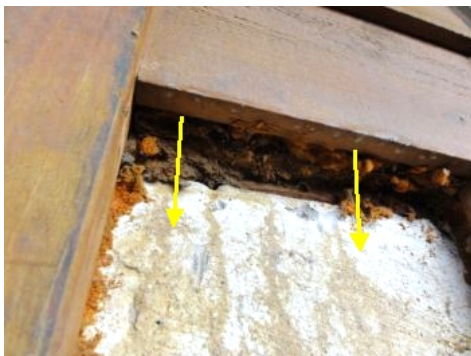
Extend siding or flash to protect sill plate.
