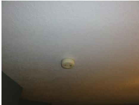
Bedroom smoke detectors lights were active, but didn't respond when pressed.
