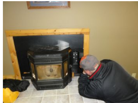
Pellet stove would not activate at controls.
