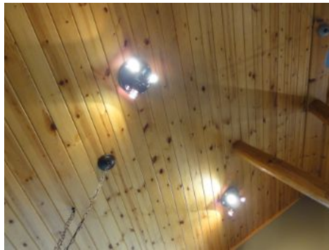
T&G knotty pine planks at vaulted ceilings.
