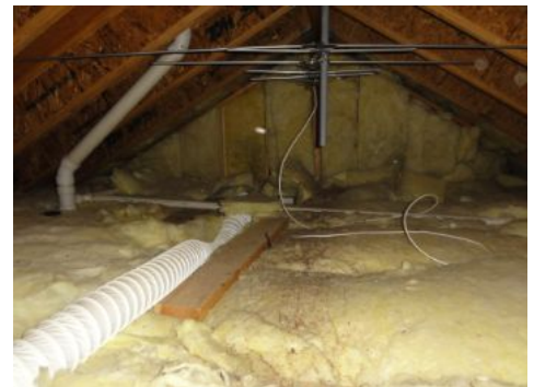
Well-insulated attic where observable.
