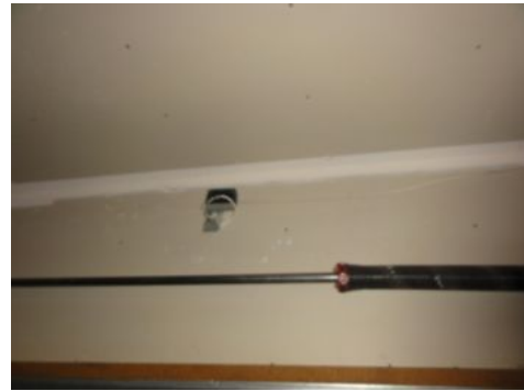
Safety feature is improperly mounted near garage ceiling, possibly for later installation.
