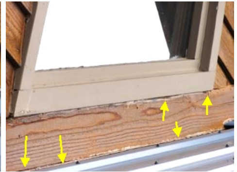
Example caulking maintenance.
