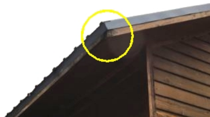
Fascia area showing wear. Monitor, some maintenance needed soon.
